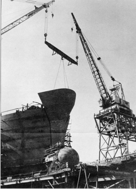
5.3: Placement of the ship's prow by two 50-ton gantry cranes on No. 8 Shipway. SSHS: 709_01_1_2r 5
