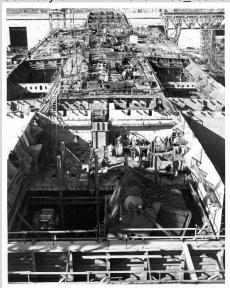
Photo showing the 'cab' of the 'Barge Crane (626\_34\_034) had been relocated to the deck of the 'Potts' to aid in the construction and free up time for the two 50-ton R-25 gantry cranes servicing No. 6 Shipway and the two 92-foot R-25 gantry cranes that service both No.6 and No. 8 Shipway. Courtesy of HML: 74.319.2186 resize
