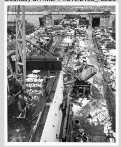
Photo showing stern of the ship with 6-Way aft gantry crane on the left and 92-aft gantry crane on the right. Note the cab on the upper trolley rail assembly that permits this crane to service both No.6 and No.8 Shipways.
