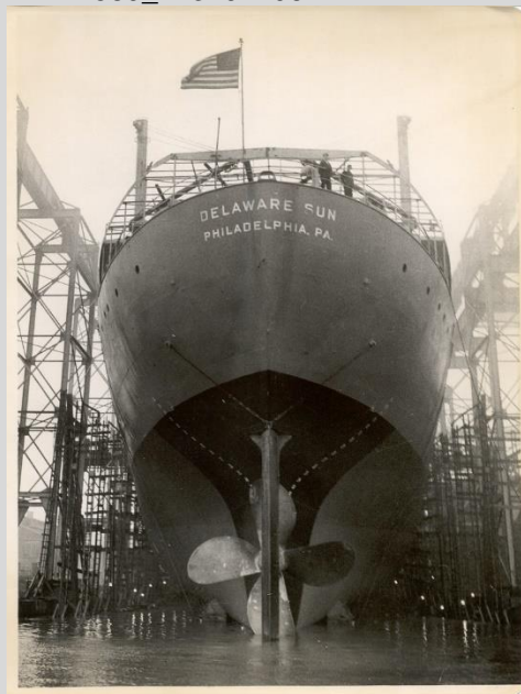
3.3: Stern view, pre-launch photo showing 22' diameter propeller Photo Courtesy of Hagley Museum and Library HML: 589_743191106r
