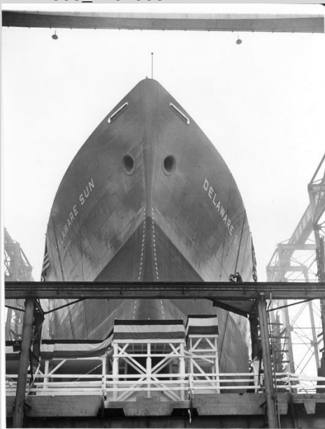
3.1: Pre-launch photo showing ship on No.1 Shipway with launching platform Photo Courtesy of Hagley Museum and Library HML: 588_74319067r
