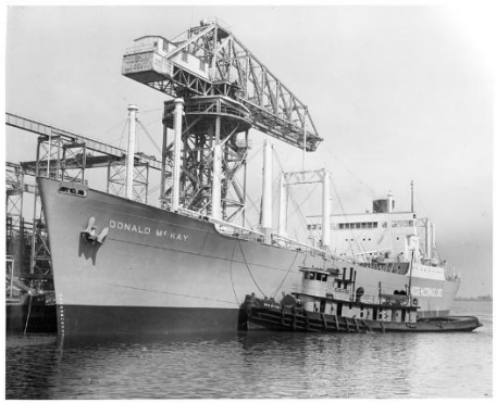
5.3 Photo taken of Sun Ship's CY 'Outfitting Basin' showing the 'DONALD MCKAY' H-175 at 1-Pier with 100 Ton lifting capacity 'Hammerhead Crane' and the Atlantic Tug 'Van DYKE 3'. Photo ID: 74319244 7
