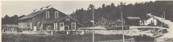
A typical pumping station on a gas pipe line in West Virginia
