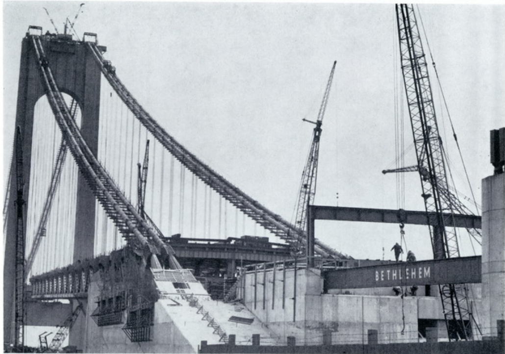
BETHLEHEM STEEL GOT THIS SHOT of steel being erected for final span at western anchorage of Verrazano-Narrows bridge on Staten Island. It also included fine view of cable saddles with strands emerging to fasten to anchor bars buried in concrete in foreground. Cable saddles and anchor bars were our contribution to this longest suspension bridge in the world. We are obliged to Bethlehem for permission to use photo.
