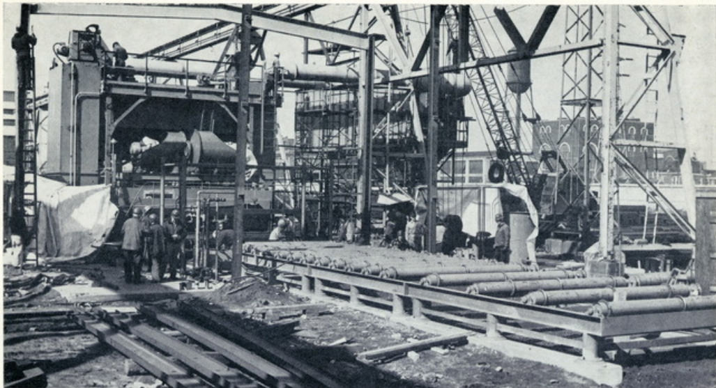
THIS APPARATUS WILL GIVE STEEL SHEETS revolving door treatment (you know — the old hag goes in and beautiful blonde comes out). On far side is platform like one in foreground. Crane lays sheet on that one. When it comes out on this side all rust has been removed and it is painted. Rust is removed by shot pelting it under pressure.
