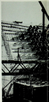
FORMS WERE REMOVED FROM SPACING AND IN PLACE INSTEAD OF ONE AS IN LEFT PHOTO. (When it will have several inches until only ready to be pulled and concrete again with the shows with 44 feet formed in concrete structure will be finished will be put in
