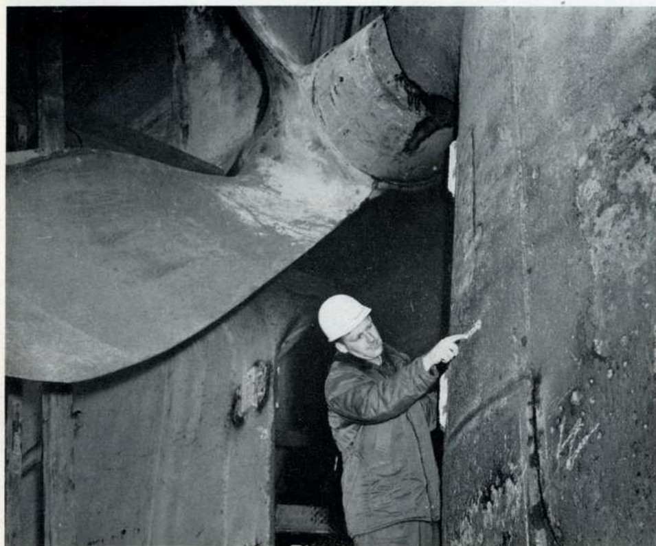
LIEUT. ROBERT F. EWELS, U.S.C.G., a hull inspector attached to Marine Inspection Office in Philadelphia, takes look at rudder of Sun Mercury as she lays in drydock #2 for annual inspection and repainting. Lieut. Ewels is responsible for certifying to Coast Guard that hulls of all ships he inspects are seaworthy.
