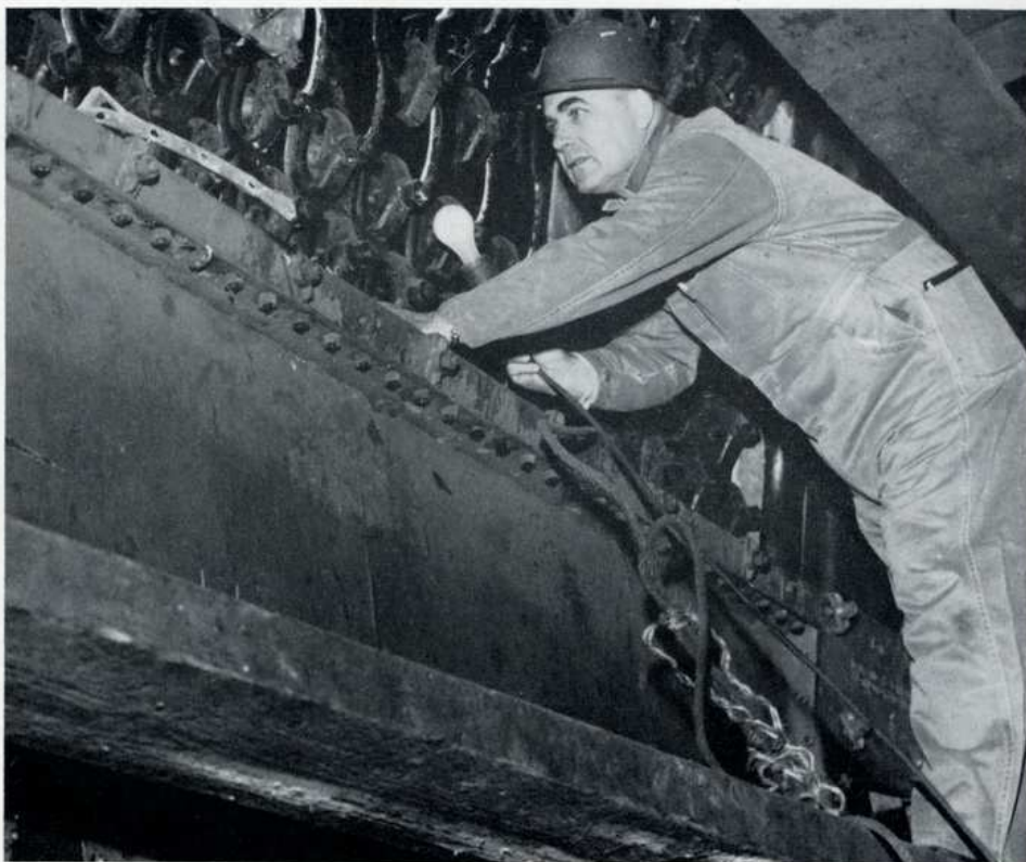
THERE WILL BE NO TROUBLE with leaking tubes in boilers after ships get to sea if Chief Machinist Warrant Officer John Chartuck, U.S.C.G., boiler inspector attached to Marine Inspection Office in Philadelphia, has been inspector on the job. Here he goes over a boiler which has been repaired in Sun Ship boiler shop prior to giving it his seal of approval.
