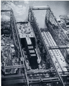
HULL 808, for the Atlantic Refining Company, in No. 2 Shipway.
