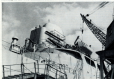
Engineering for the Sun Oil Co. rig, showing the rig from the side of the structure.
