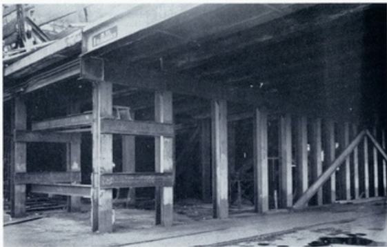
DO YOU KNOW what is going on under No. 2 shipway?
