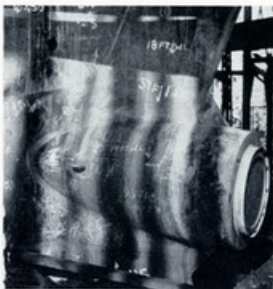
Fig. 4 — CLOSE UP OF DETAILS around boss casting (welded in Hull 598).
