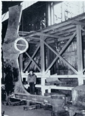
Fig. 1 — COMPLETED WELDED STERN FRAME in 47 Shop. (Next operation Stress Relieving.)
