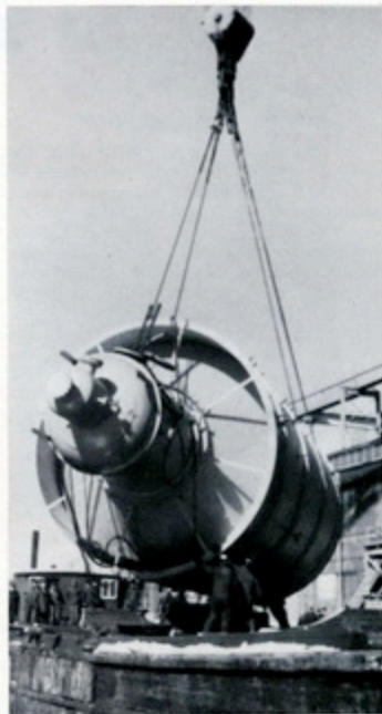
THIS HUGE OIL REFINERY TOWER was brought through the Boiler Shop door with inches to spare, and out on #5 pier. The hammerhead crane transfers it to the barge.
