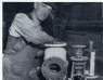
4 - WALTER WELLS , Diesel mechanic Wells with 20 years service is shown grinding the ribs of a turbine regulating valve.
