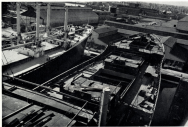
WARNING — CRIMINALS AND THIEVES — In the photo, to the left, under the right eye, and to the right, the other 14 show the getting, pulling, tacking of the frame plates on the "backbone" of the structure and the steel "girders" (main beams), making the structure and covering. Ripping, chipping, chiseling, tapping, etc., blocks (bricks), long pipes (cables) cut down through the deck and steel beams.
