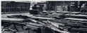
THE BELT is very long—two miles to be pulled up the last conveyor section of the mill. It is made of heavy-duty metal plates.
