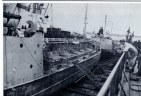
THEY'VE BUILT (LEFT) ONE OF THE NEW 600 TONS, each having 1,000 barrels carrying capacity, at 275 Bay Blvd. of the new four ship dock. The bottom completely consisting of aluminum and steel framework and other tube grating work, were completely dismantled and reworked.
