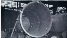
PICTURES TALK SHORE — Top — One of the tube sections for a large special condenser being hoisted out of the boiler shop for use of the oil-refining in this vicinity. Lower — A section of the shell for the same job.
