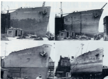
(1) — PENNSYLVANIA TON — furnace damage and general repairs.
