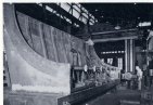
CONDENSER SECTION which was fabricated in our Shop (they being assembled in the Washmill Plant. This job required a Brown facing of wide 14" ribs and a center of 14".
