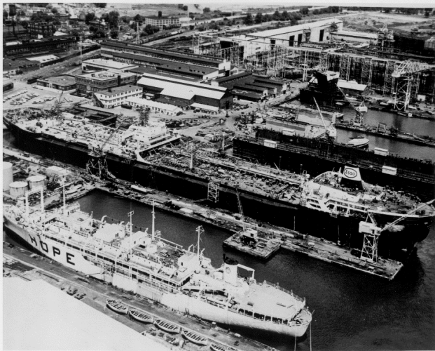
#218_04_01a Closeup of the No.3 Dry Dock extension, used to build and launch the Sun Ship 122'8-1/4" bow section and drydock outrigger at 3 Pier North
