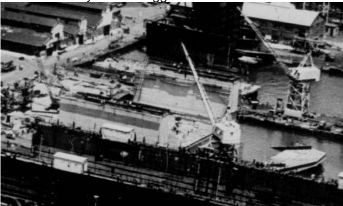
#218_04_01a Closeup of the No.3 Dry Dock extension, used to build and launch the Sun Ship 122'8-1/4" bow section and drydock outrigger at 3 Pier North
