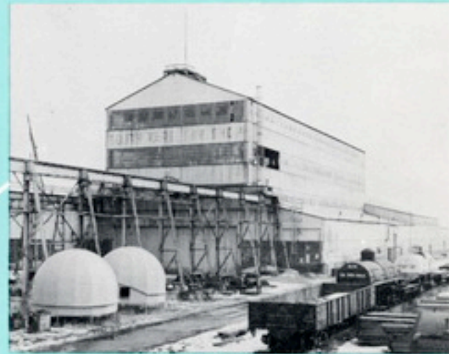
South Yard Fabricating Shop
