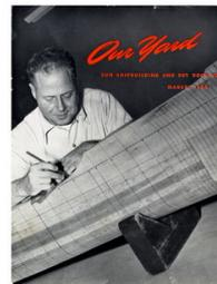
TO THE LEFT IS A PICTURE OF A DRAFTSMAN DRAWING THE LINES THAT WILL REPRESENT THE ACTUAL PLATES THAT WILL BE ORDERED FROM THE STEEL MILLS TO BUILD THE SHIP.
